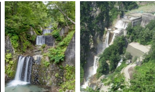
① Dorodani Sabo Dams (sediment generation control) ② Shiraiwa Sabo Dam (Sediment check)
