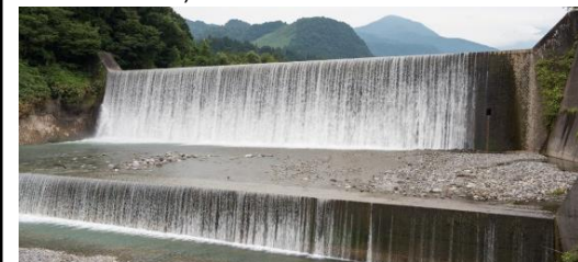
③ Hongu Sabo Dam (sediment storage and adjustment)
