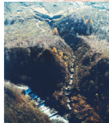
泥谷砂防堰堤
